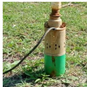
Figura 8. Bomba solar sumergible
